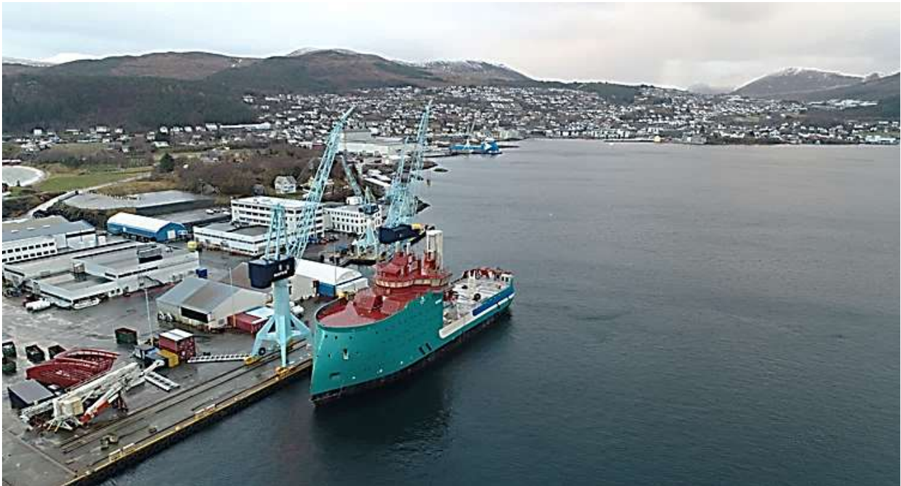
Ulstein Verft_AS, Norveška_Photo credits: Ulstein Group ASA
