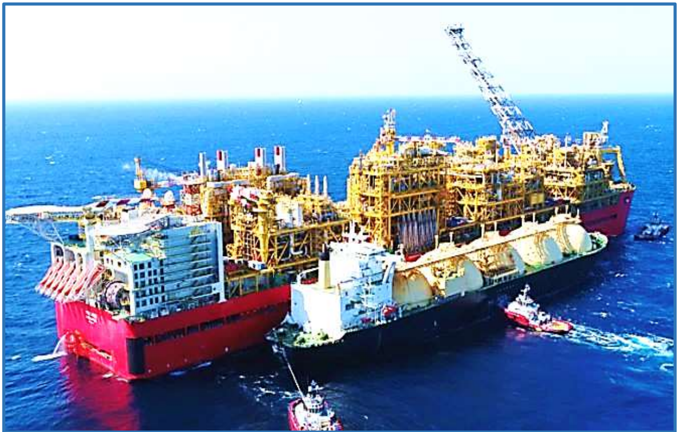
Shell 06/08/2018 uvodi plin u FLNG Prelude radi oživljavanja i ispitivanja postrojenja Photo credit: Offshore Energy Today
