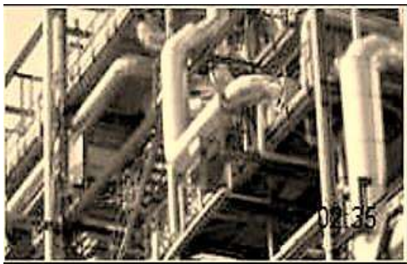
Postrojenje Beta Renewables u Crescentinu
